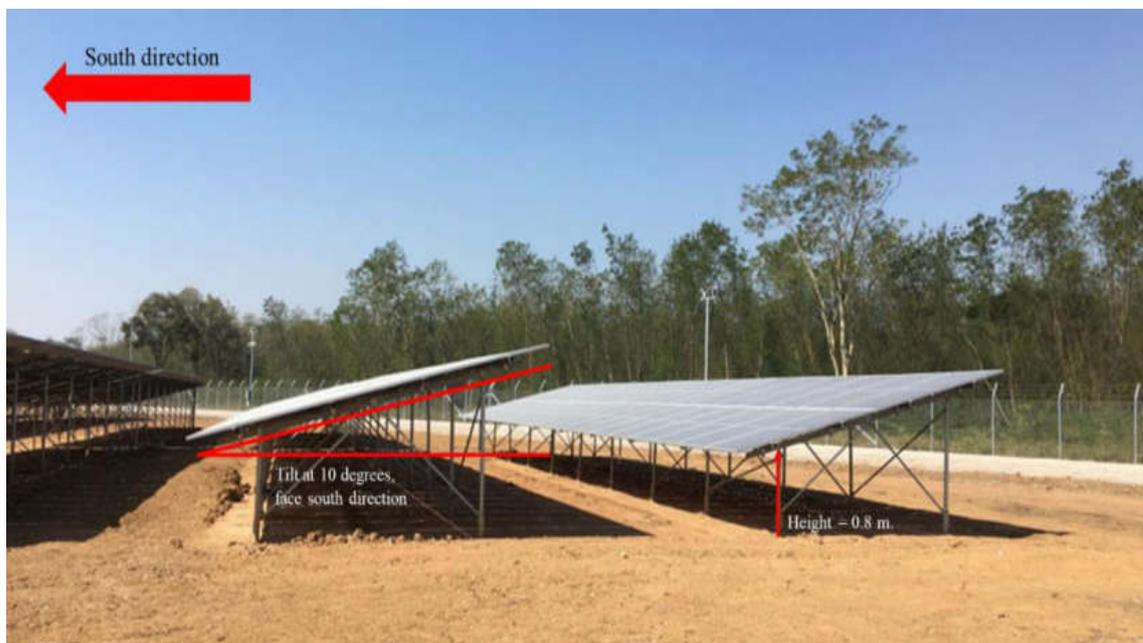
**Figure 2.2.1.2-1 Ground Mounting Structure Facing South Direction**
