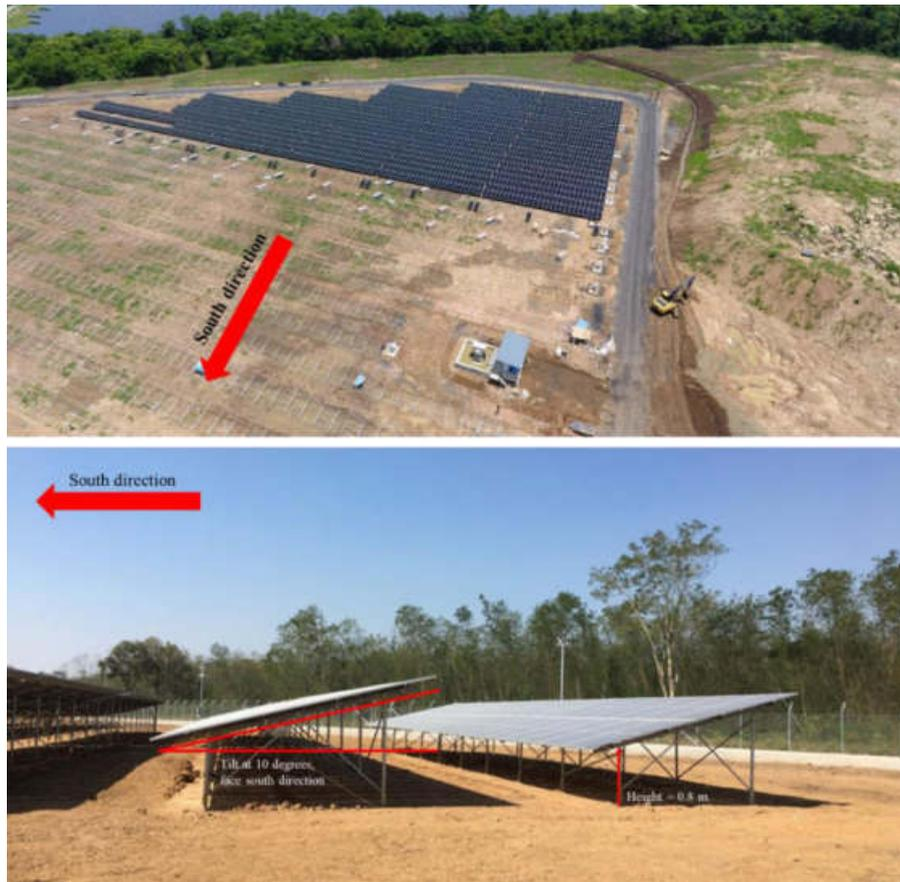
**Figure 2.4.1.1-2 Structure and Modules Installation**
