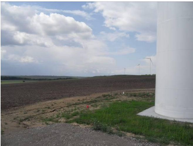
Figure 8 – View from base of turbine 7
