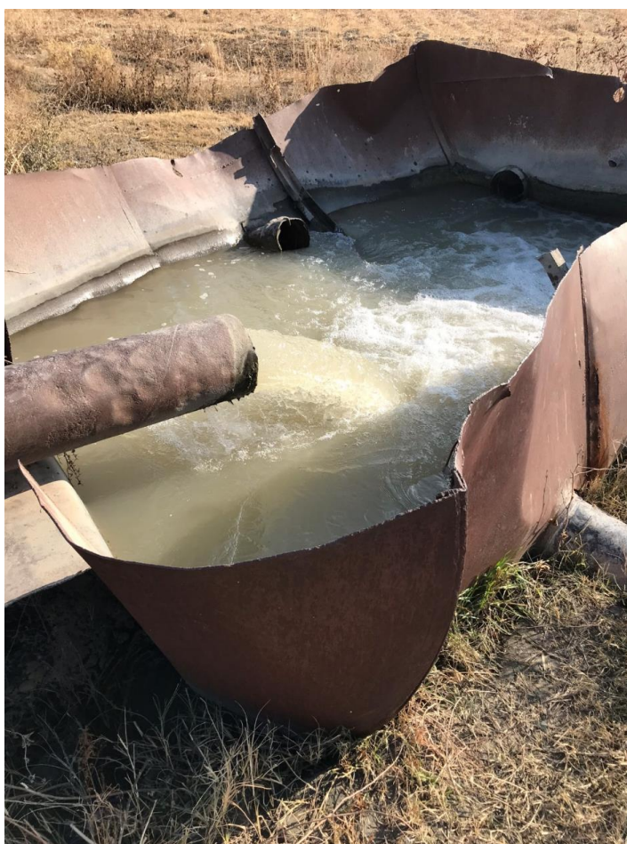
Figure 6-12. Irrigation water discharging into the irrigation system
