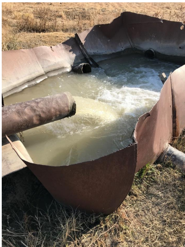
Figure 6-17. Outflow of water pipe from Zarafshan River to irrigation system
